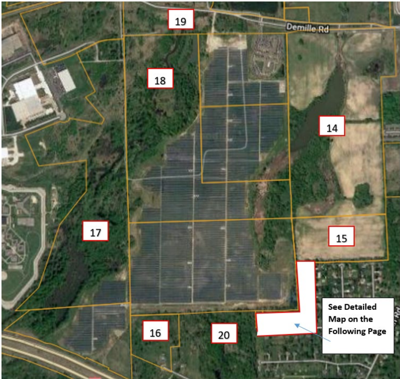
DTE's Lapeer Solar Projects - Demille Adjoining Properties
