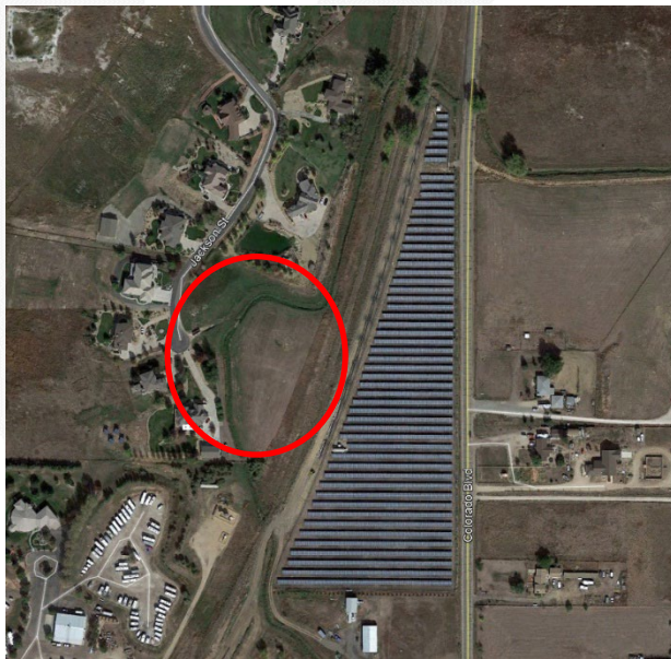
Brighton PV Solar, Adams County, CO June 2016
