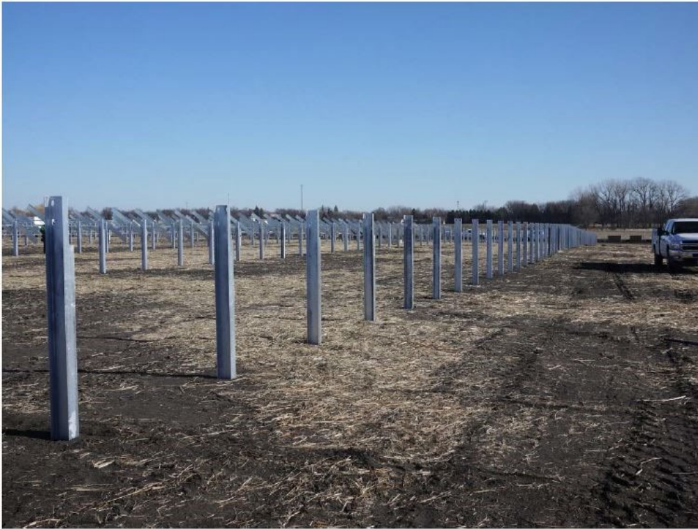
Figure 3.1.1-3 Standard Steel Pier Foundations
