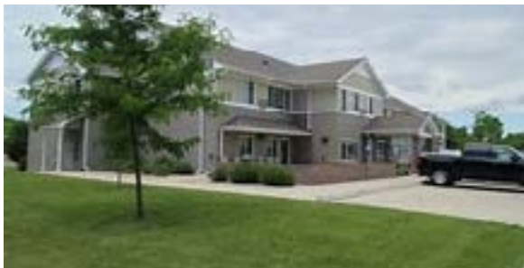
Buffalo Ridge Apartments, Worthington
